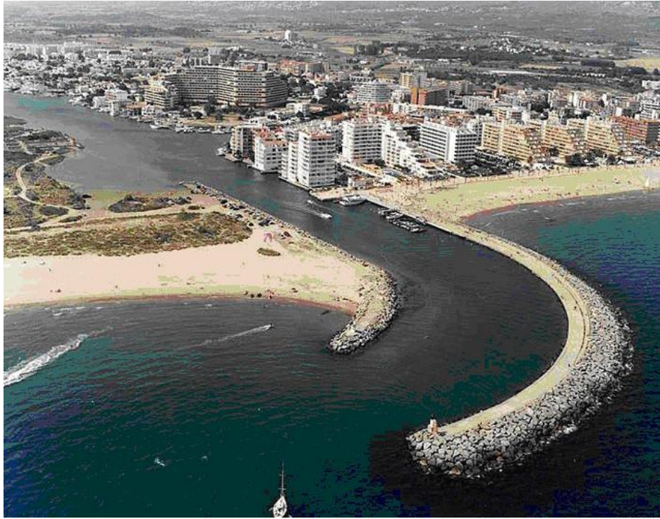
Estuary of the river Grao and Margarita. To the right in the picture you see the beach area which is the demarcated stripe of public land (Domono Publico) of the urbanization (first line on the beach) closely occupied by large buildings. In the background the Urbanization Canales de Santa Margarita in part hidden by the building „Seiscientos“
